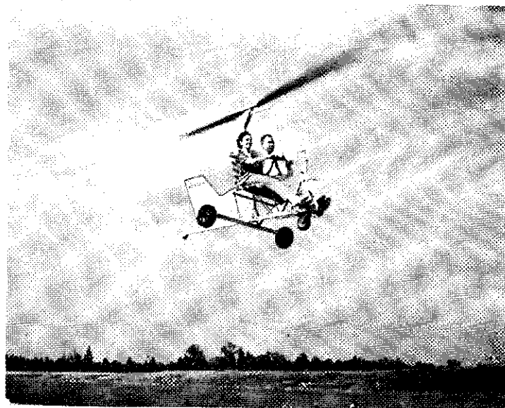
Fig. 21—The 8-8 Gyro-glider modified with a dual seat, lifts easily two people. Dual instruction can be profitable for both the student and the instructor, can be a lot of fun, too.
