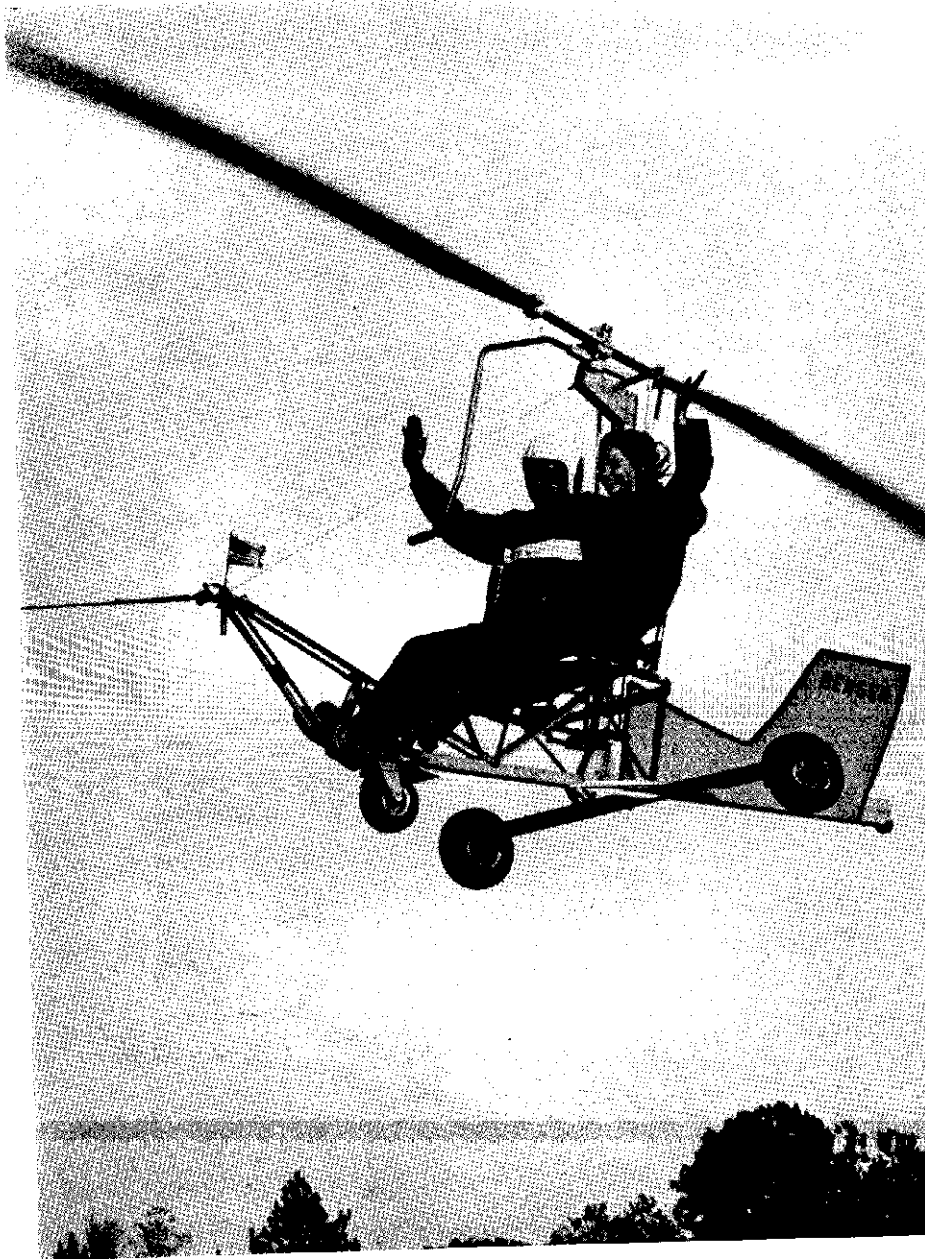
Fig. 1—Gyroglider flying can be a lot of fun when giving rides to your friends in the dual-seat convertiplane. This particular Gyroglider is equipped with both types of control stick—overhead and joystick. The machine is so easy to fly, and so that it flies hands-off all by itself.
